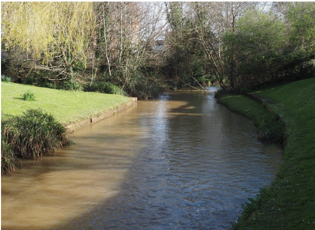
Fig. 14: Coppins Bridge, 29 th March 2024
