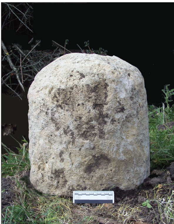
Plate H. Bembridge Limestone pier or spur-stone possibly derived from the first structural phase of Key Cottage.
