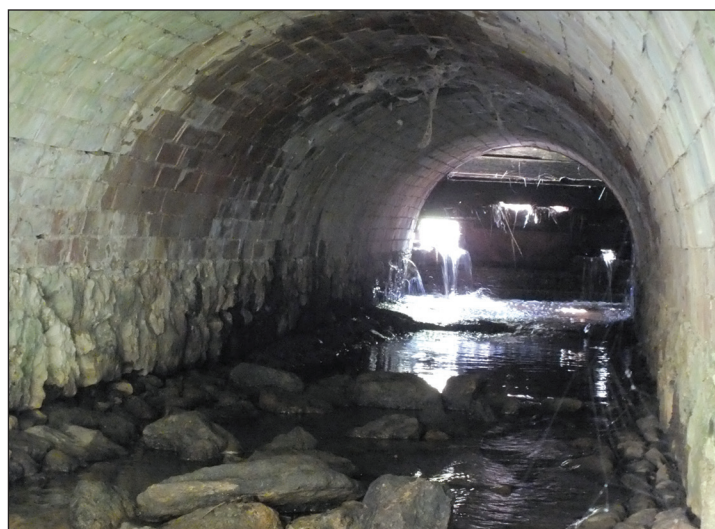
Figure 9: The stone-lined culvert beneath Quarr Road, looking south (Photo: Roger Simpson).
