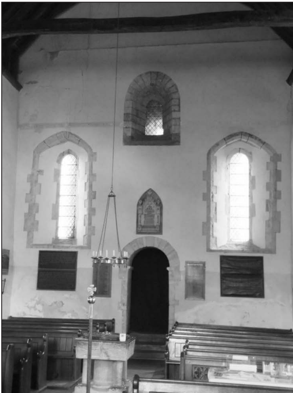
Figure 2: The western wall of the nave of Arreton church, showing the doorway and the single-splayed window above, also constructed of Quarr stone. The flanking lancet windows were inserted into the west wall of the nave in the earlier part of the thirteenth century.
