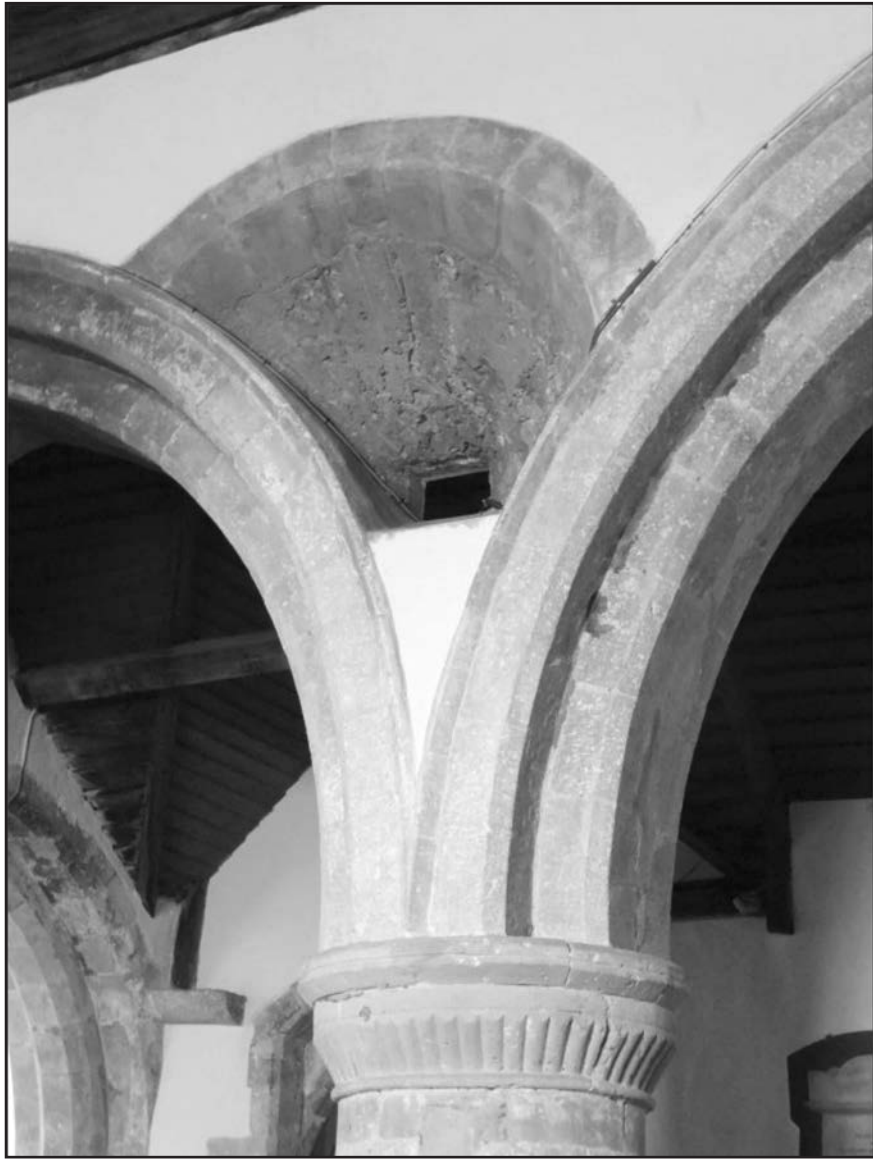
Figure 6: The arcade on the south side of the nave in St Mary's church, Carisbrooke was constructed in the Transitional Norman style of the late twelfth century. The photograph shows one of two examples here of single-splayed round-headed windows which were partially cut away with the insertion of the arcade into this wall. These two windows would appear to be broadly contemporary with the single-splayed windows in Arreton church. St Mary's was one of the Island churches given to the Norman abbey of Lyre by William fitzOsbern c.1070.
