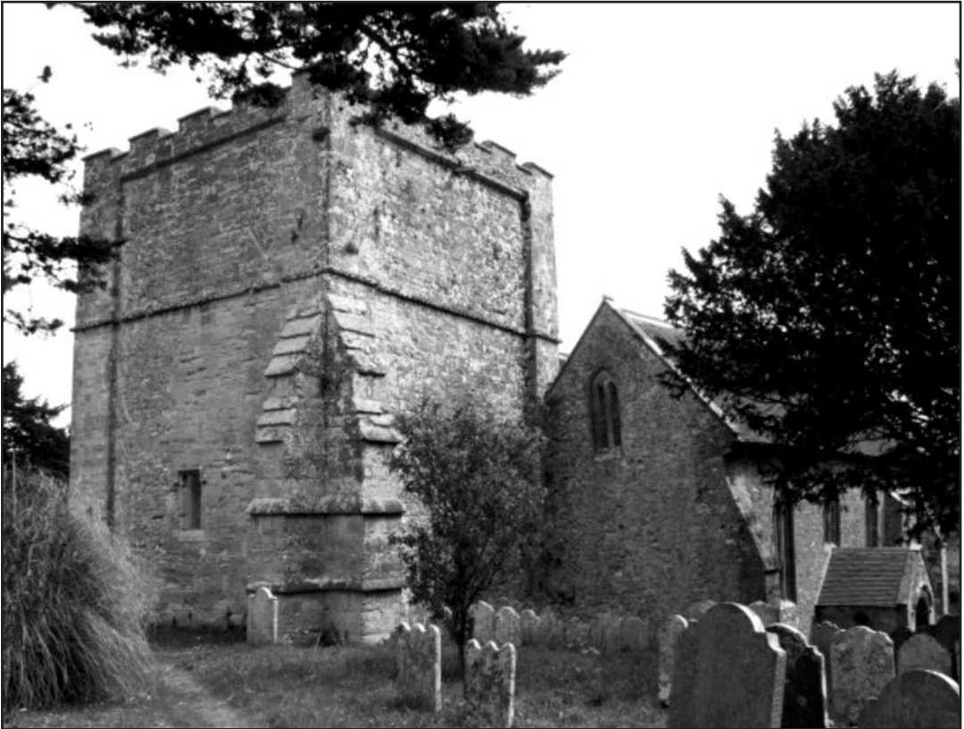
Figure 9: Shalfleet church from the south-west. Domesday Book records “a church” here. The massive western tower with its billet-moulded string course would appear to have been constructed in the early Norman period. The north doorway of the nave with its fine tympanum can be dated to c. 1150.
