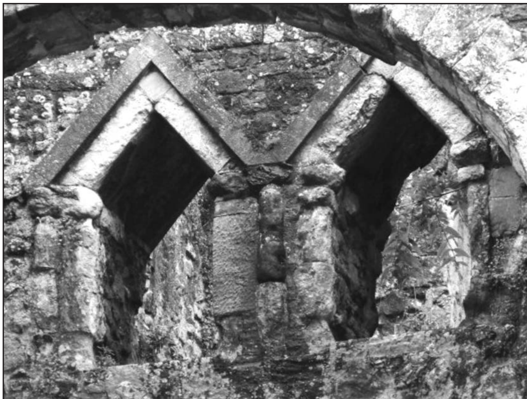
Figure 3: Two triangular headed openings in the gatehouse of Rougemont Castle, Exeter. The gatehouse was probably constructed in 1068-9 and incorporates a combination of Anglo-Saxon workmanship and post-conquest Norman architectural features.
