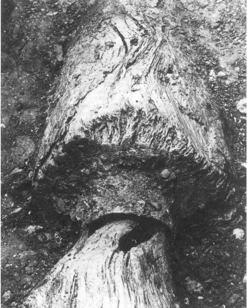
Plate 1. The first piped-water system at Newport, Isle of Wight. Section of the elm water main with lead collar junction, laid 1617–1623. (Newport High Street 1980) Photographs Les Allan.
