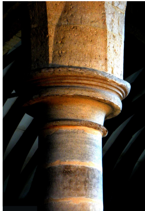
Fig. 18: Purbeck Marble capital and 'drum' components in a 13 th century nave pier in Shalfleet church.
